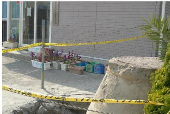
appeared in the ground, water pipes broke, and a manhole in front of the building popped up from the ground (please see the picture above).
